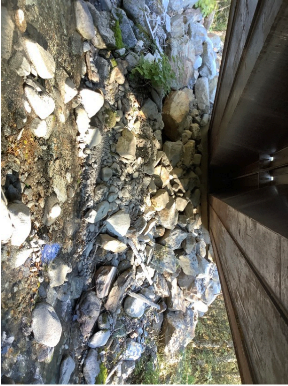
Left Bank Abutment when facing downstream
